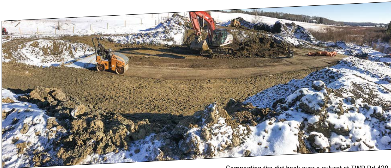
Compacting the dirt back over a culvert at TWP Rd 420, over the East Lobstick Creek (NE-34-41-6-W5)
