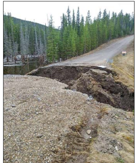
Washout on Wapiabi Road (Northwest of Nordegg)
